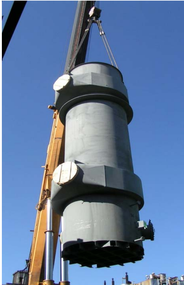
Fig. 15 Erection of Recuperation Heat Exchanger
