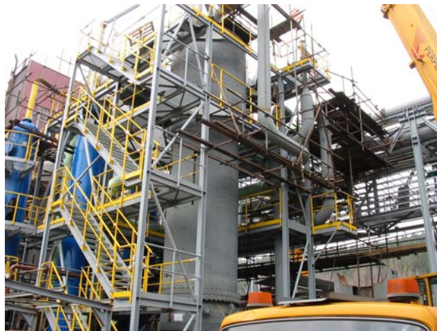
Fig. 16 Erection of Heat Exchanger Set of Crude Gas Cooling Unit
